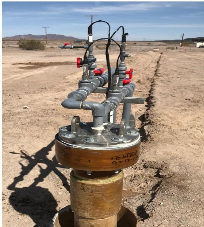
**Figure 1: Commercial Scale production well head at Fort Cady being used for pilot plant testworks**
